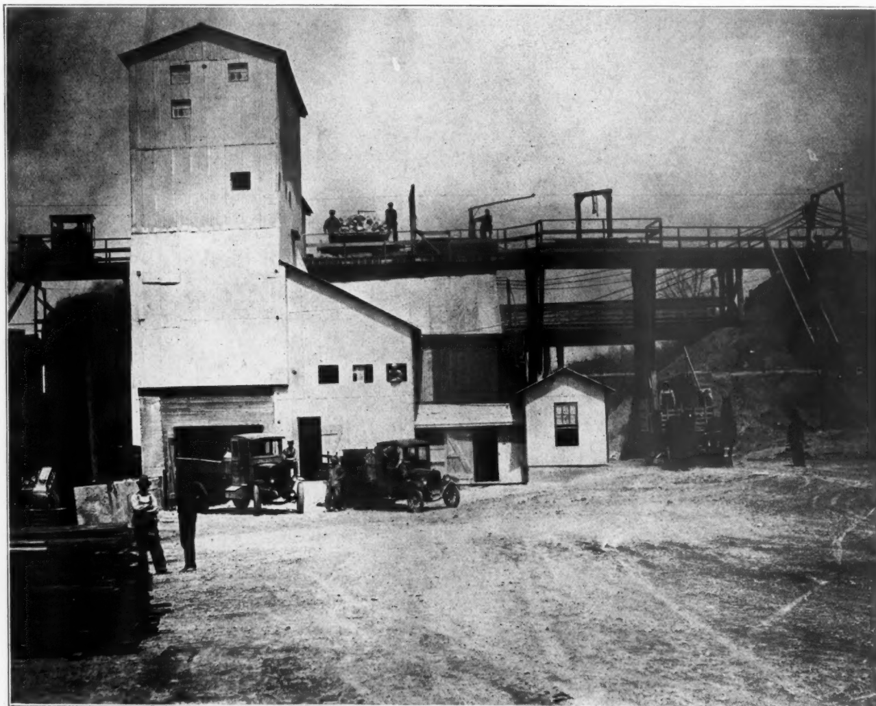
General View of Agstone Mill
